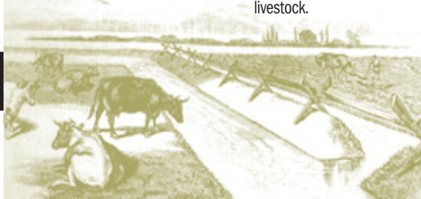
American Indians in the desert Southwest captured water in basins and created canals to irrigate their crops. Settlers who came later would use similar techniques, such as wooden check gates, to divert water to crops and livestock.
