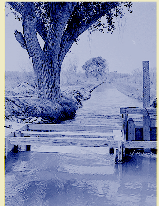
American Indians in the desert Southwest captured water in basins and created canals to irrigate their crops. Settlers who came later would use similar techniques, such as wooden check gates, to divert water to crops and livestock.
