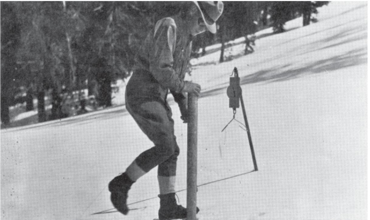
The snow is measured by a special metal tube. The men thrust it down through the crusted snow just as you see in the picture on the opposite page. They do this to find out exactly how deep the snow is. Then they weigh the snow that is inside the metal tube just as you see the man doing in the picture below. From this information they can tell how much water the snow will make. They can then find out how much water to expect the next summer for our crops and for use in our cities and towns.
