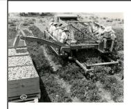
The mechanical tomato harvester, used to harvest, sort, and load tomatoes, was developed.
