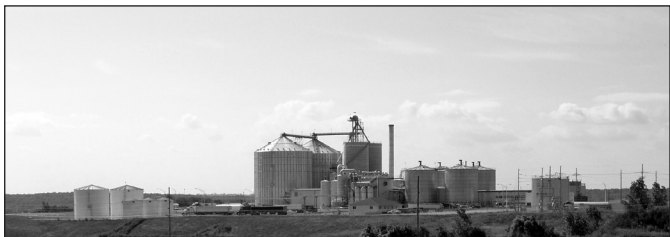
East Kansas Agri-Energy Ethanol Plant, Garnett
